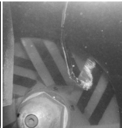
Fig. 6.38. Vortex rope generated in the inlet; the vortex is cut by the blades
